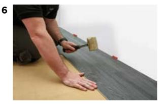
Once you have positioned each "short end" into place use a rubber mallet to tap the drop lock system into action. This should be done on every short end joint. The long ends do not require any additional force to lock into position.
