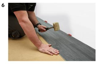
To start the 2nd row, position the drop lock joint of the panel over the joint of the panel in the 1st row and tap into place using a rubber mallet. Again, take care to ensure the joints are perfectly aligned before tapping into place. Continue the 2nd row by angling the tongue of the 2nd panel into the groove of the 1st panel and tapping the drop lock joint into the adjacent panel of the 1st row. Repeat the process until all rows are installed.
