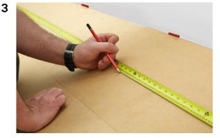
Measure from wall to wall and ensure that you start installing in a logical place to minimise any cuts across the panels to the perimeter of the installation. Mark a "starting line" on the floor with your pencil. Ensure that you include the 5mm expansion gap when measuring.
