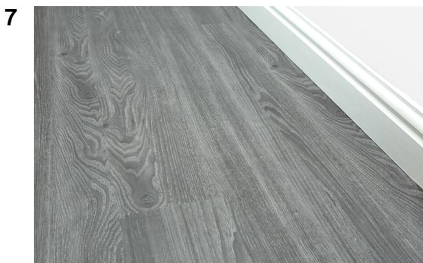
Now your floor is fully installed, you can replace your skirting boards. Be careful not to fully trap the flooring as it needs to be able to expand and contract freely. Usually 1-2mm is enough to allow this to happen. If you left the skirting boards on, then use Scotia beading to cover your 5mm expansion gap. Never use any type of filler to cover your expansion gap.
