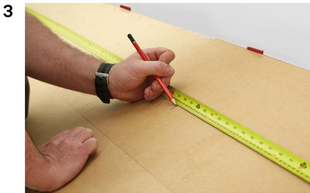
Measure from wall to wall and ensure that you start installing in a logical place to minimise any cut planks to the perimeter of the installation. Mark a “starting line” on the floor with your pencil. Ensure that you include the 5mm expansion gap when measuring. More information in the detailed fitting instructions in each box.
