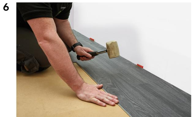
Once you have positioned each “short end” into place, gently tap the top surface of the plank using a rubber mallet (from a height of approx 10cm above the surface) to engage locking system. The surfaces of the planks should be perfectly flush after tapping down. Do not use extra force and never use a solid tool such as a metal hammer as this could cause damage to the joint.
