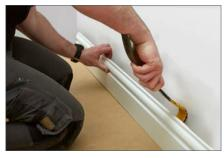
A 5mm expansion gap is needed around the entire perimeter of the flooring. You may wish to remove the skirting boards and replace after installation or use Scotia beading to cover the expansion gap. In this instance we have removed the skirting boards.
