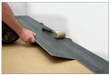
Start the installation by angling each plank into the click locking system along the long ends and then lay each plank flat to the floor. The long ends have a click lock system to hold each plank in place. The short ends have a drop lock system. More details in the detailed fitting instructions.
