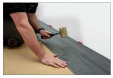
Once you have positioned each "short end" into place use a rubber mallet to tap the drop lock system into action. This should be done on every short end joint. The long ends do not require any additional force to lock into position.
