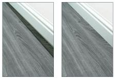
Now your floor is fully installed, you can replace your skirting boards. Be careful not to fully trap the flooring as it needs to be able to expand and contract freely. Usually 1-2mm is enough to allow this to happen. If you left the skirting boards on, then use Scotia beading to cover your Smm expansion gap. Never use any type of filler to cover your expansion gap.
